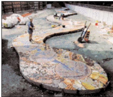
On site installation at Darling Harbour, Sydney
