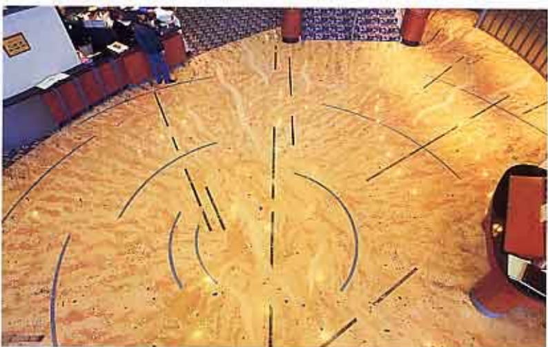
Terrazzo floor, lobby of the Campbelltown Catholic Club
