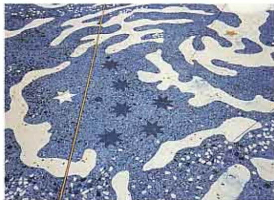
Detail of terrazzo floor works
