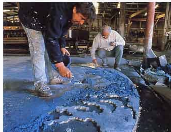
David Humphries working on a terrazzo installation
