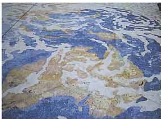
Detail of terrazzo floor works
