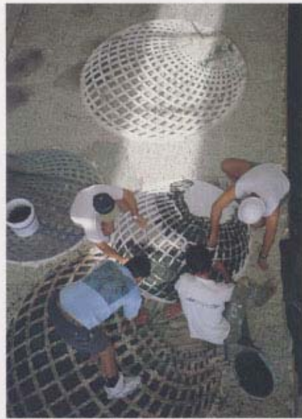
Installation of water-jet-cut marble inlay for terrazzo floor
