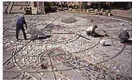
Installation of terrazzo mosaic, Celebration Place, Robina
