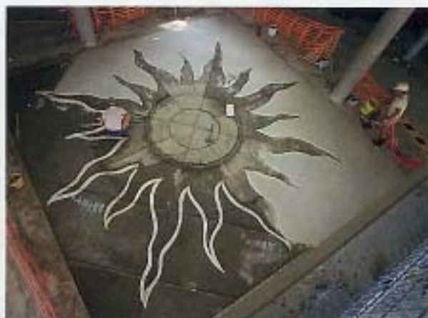
Right: The 'Sun Floor' being laid, showing polystyrene templates in position
