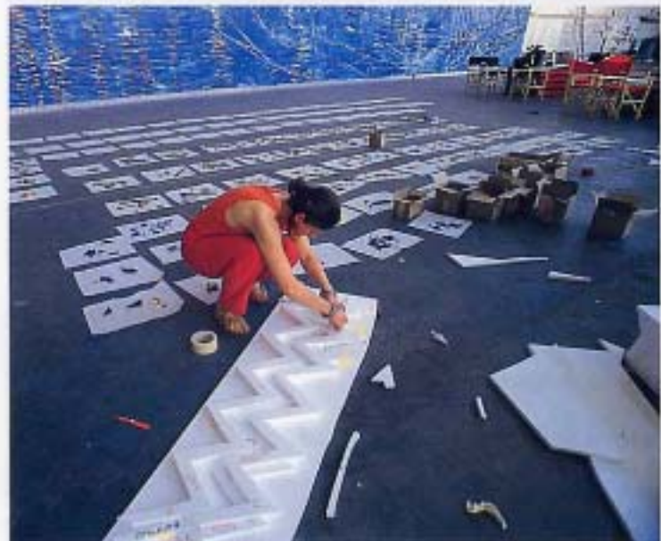
Positioning polystyrene templates for terrazzo design by Thancoupie
